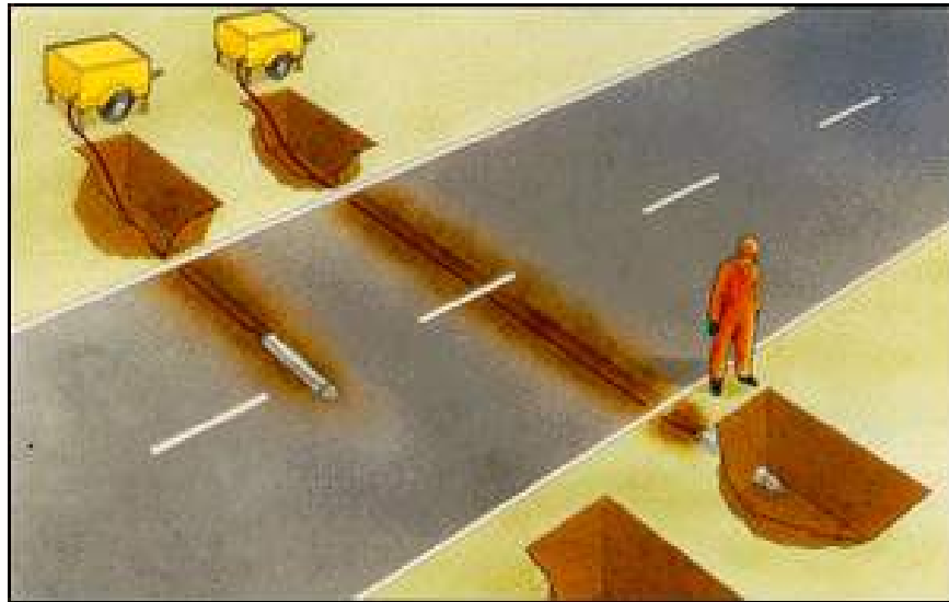
Figure 2.3.1 Impact moling
